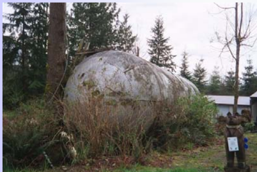
Poorly maintained reservoir Credit: Rural Community Assistance Corporation
