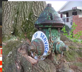
An out of service fire hydrant in DC
