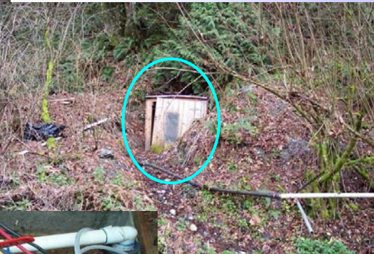
Spring Box with open access
