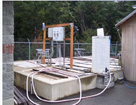
Small wastewater treatment plant
