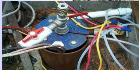
Wellhead that needs to be replaced
