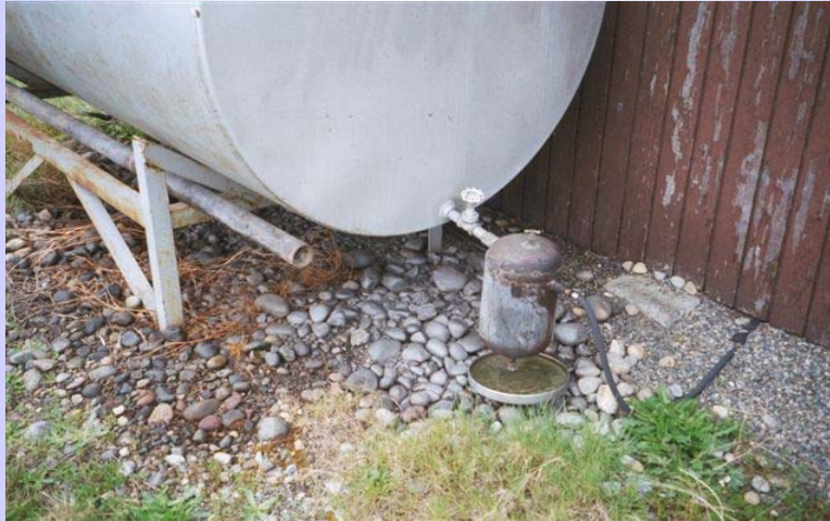
Fuel tank leaking diesel next to wellhead
