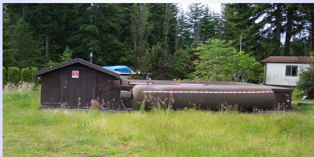
Small system wellhead with hydrotank
