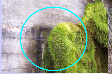
Leaking reservoir wall
