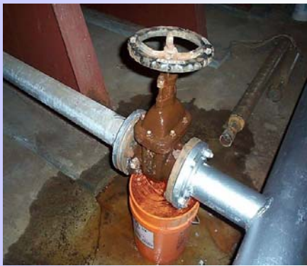
Leaking valve Credit: Rural Community Assistance Corporation
