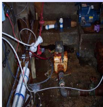
Failed booster pump results in well house flooding
