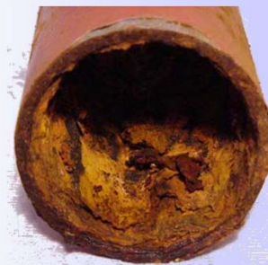
Rusted iron water pipe Credit: Timothy Ford, Montana State University
